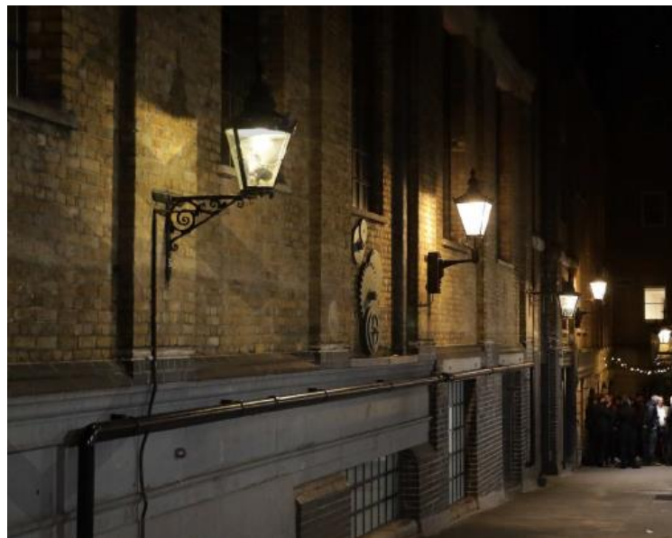
Bull inn Court, gas in foreground, trial replica LED in background
